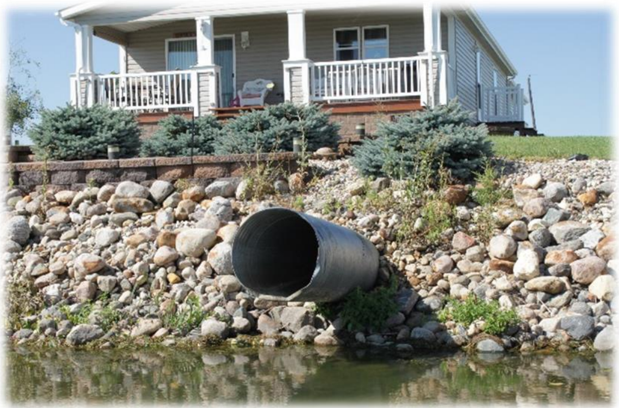
Figure 14. Drainage Culvert located in Block's Bay
